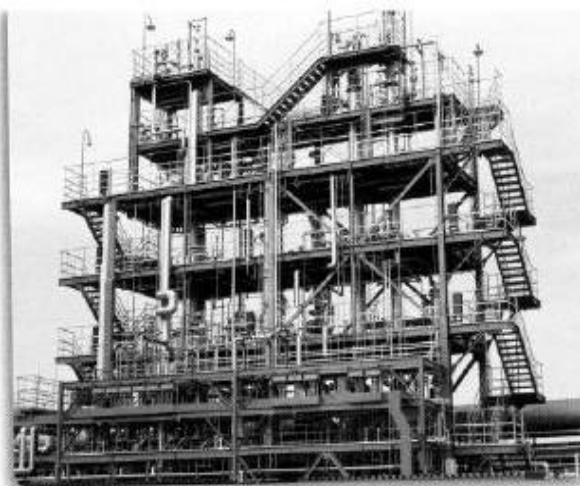
CO 2 -methanol plant.
